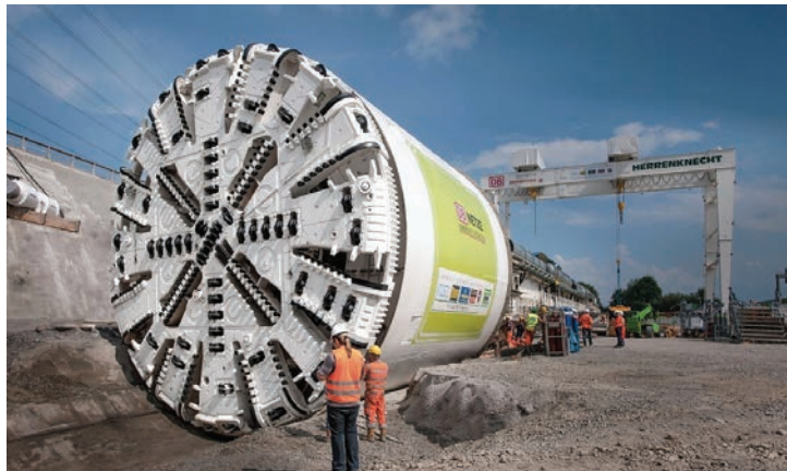
Photo courtesy of Herrenknecht AG
